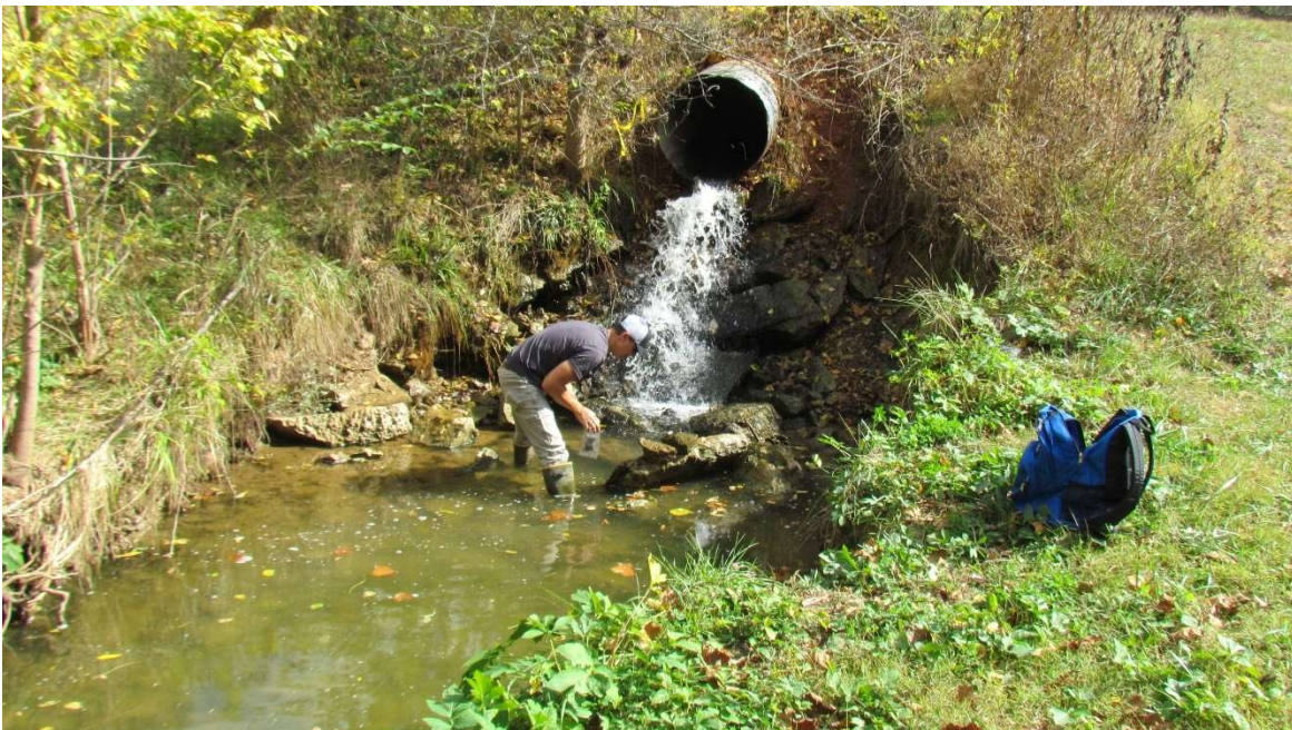
Figure 2. Discharge from corrugated pipe in HFP Spring Lake.
