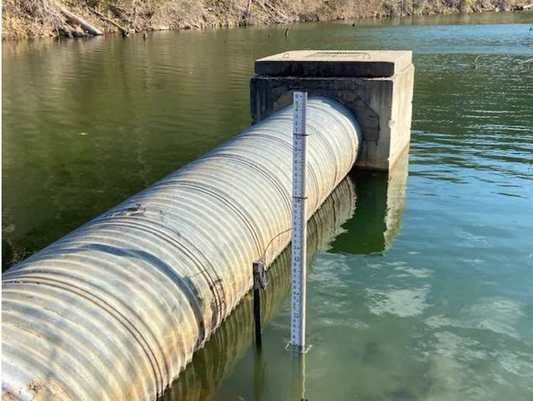
Figure 1. Location of water level logger and staff gauge near the HFP Spring Lake outflow structure.
